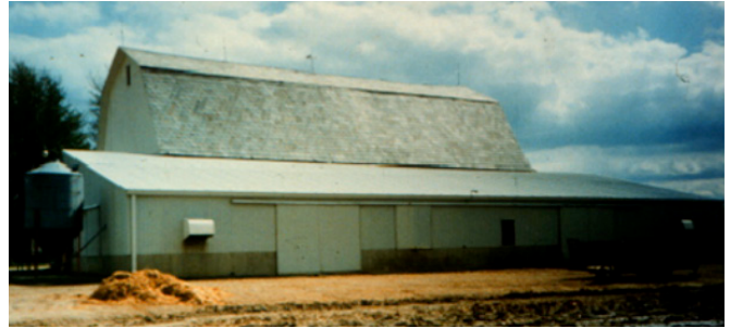
Figure 2: Dean Genter's rehabilitated barn with new attached side shed. Archbold, Ohio.
