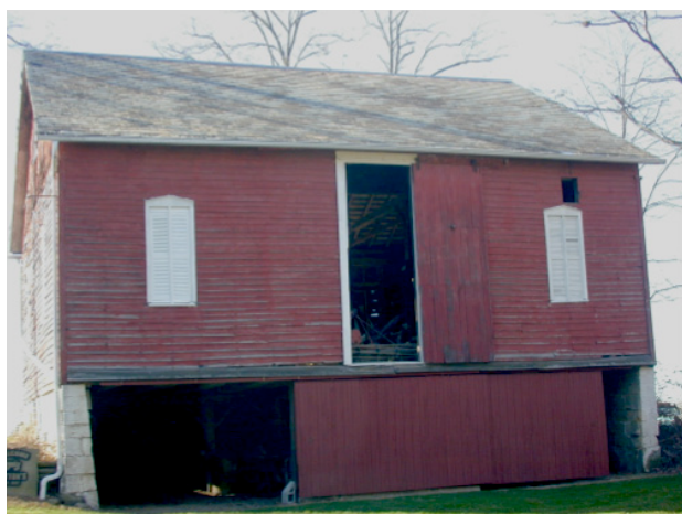
Figure 1: Raised basement three bay threshing barn near Alliance, Ohio.
